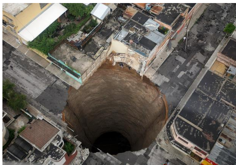
Figure 6- 2010 Guatemala City sinkhole. Photograph courtesy of Paulo Raquec (2010).
